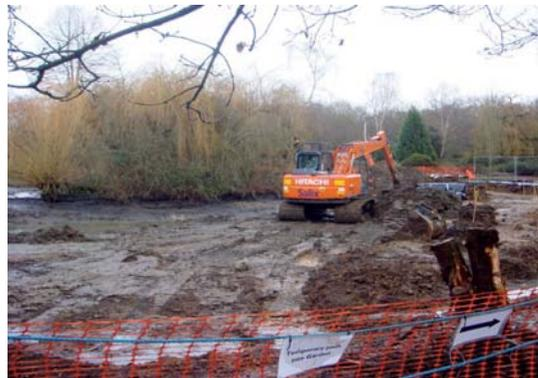
The restoration work on the ponds in Isabella Plantation started on schedule in early January, but the delivery lorries and excavation equipment quickly churned up the waterlogged ground (*see below left*), and the contractors had to bring in a cover of gravel, which will have to be removed (at their expense) once the work is finished. The Isabella ponds and streams work should be completed by the time you read this.
