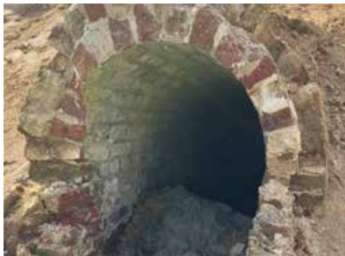
The damaged culvert dating from 1746
